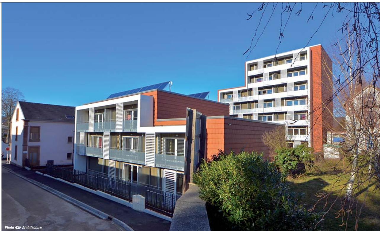
Photo ASP Architecture
