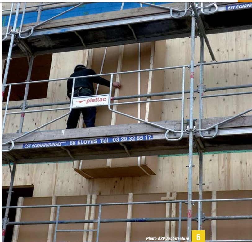
Photo ASP Architecture 6
